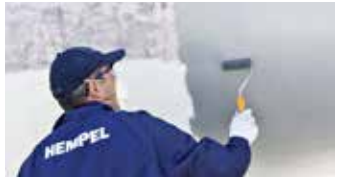
Apply Hempel's Underwater Primer onto prepared surface
