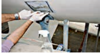
Wet scrape to remove old antifouling
