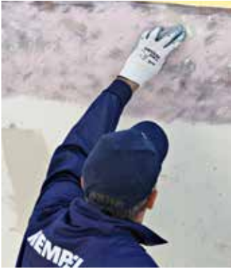
Fill along boottop
