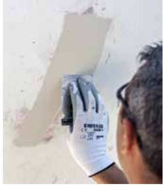
Fairing any defects
