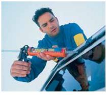
It is essential that the glass meet all the demands and standards required for the intended application. For insulation glass, total bonding consistency must be ensured through the complete use of Sikaflex® adhesives for all the installation, i.e. no silicones. The polyurethane adhesive bond face must also be protected against UV radiation. This may be achieved by several means:
