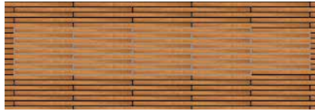
3. Embedded new planks
