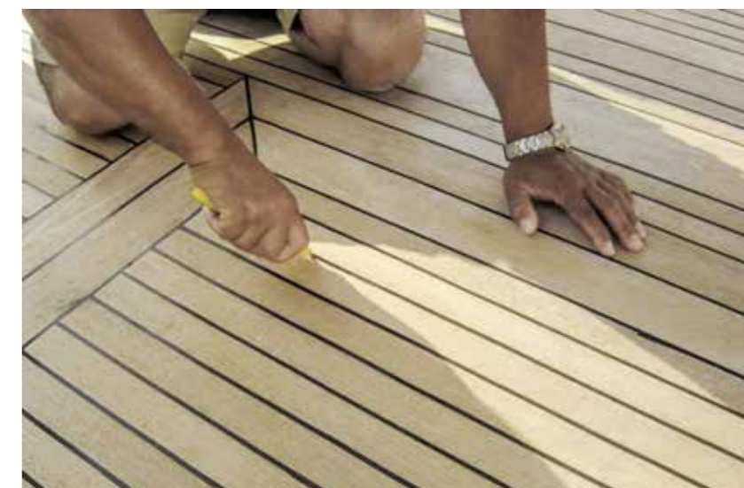
Fig. 60 Using a craft knife to cut along the part of the joint to be removed
