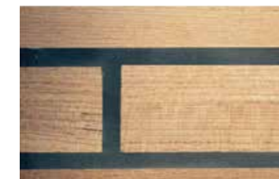
Fig. 55 New teak deck
