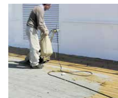
Fig. 46 Sanding the deck
