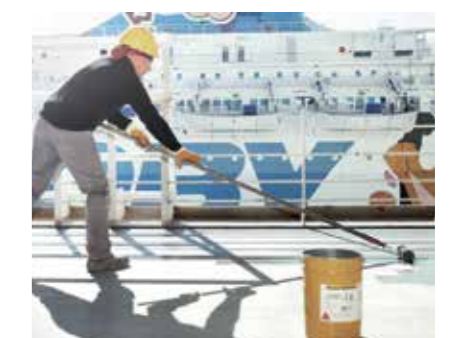
Fig. 29 Applying SikaCor® ZP Primer with a roller
