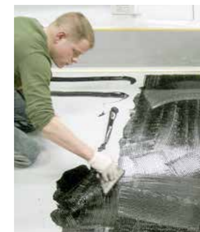
Fig. 81 Application of Sikaflex®-298
