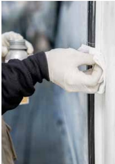
Fig. 99 Pre-treatment of the ceramic ink area with Sika® Aktivator-100
