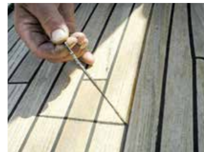
Fig. 71 A triangular cut of the old caulking being removed manually
