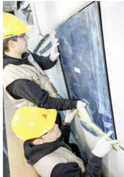
Fig. 101 The window is fitted
