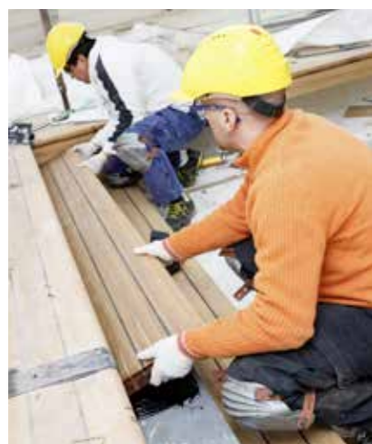
Fig. 39 Putting down the decking
