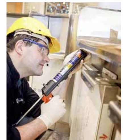
Fig. 90 Application of Sikaflex®-291i
