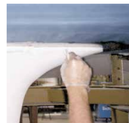
Fig. 107 The joint is tooled off and finished
