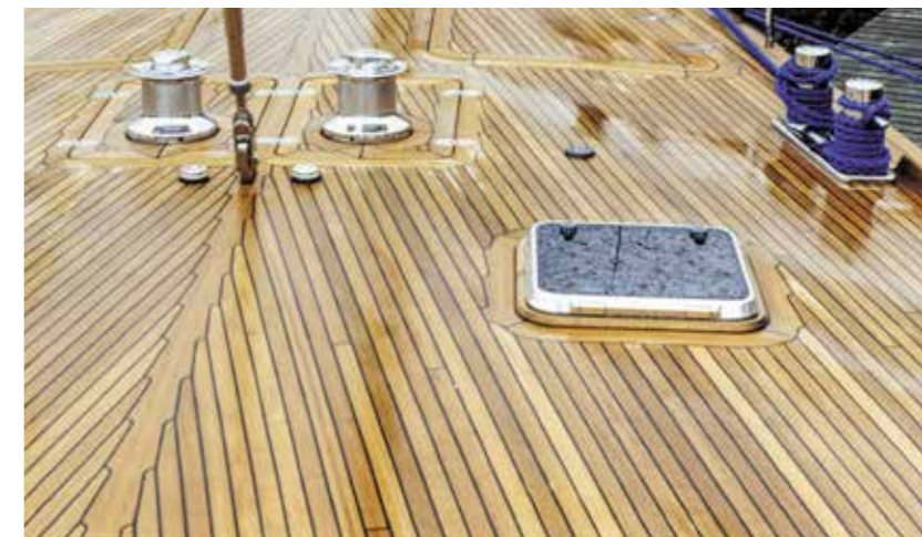
Fig. 56 Keep decks looking like new by using the appropriate maintenance products
