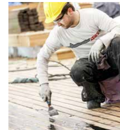
Fig. 45 Compressing Sikaflex®-290 DC PRO with a spatula
