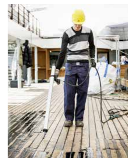
Fig. 43 Applying Sikaflex®-290 DC PRO
