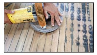
**16.** When caulking has cured, sand surface of deck to remove excess caulking using 80-100 grit sandpaper with a soft pad on a grinder.
