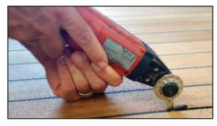
**3.** Other more precise electrical tools can be used to cut out the old caulking, and in some instances, deepen the seams.
