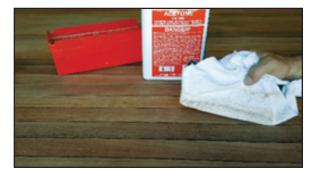
**9.** Thoroughly clean and de-oil the seams by wrapping a clean rag around a 6" putty knife (or similar flat surface). Moisten rag with acetone. Use a back and forth motion, rotating the rag frequently. Let acetone dry, then caulk immediately after applying bond breaker tape (fine line plastic tape).
