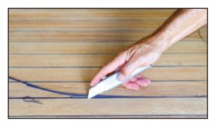
1. Old or damaged caulking can be removed with a razor knife, taking care not to damage the wood fiber.
