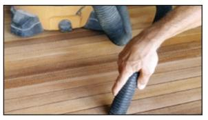
**8.** Prior to de-oiling, the dust particles should be removed by vacuum or compressed air.
