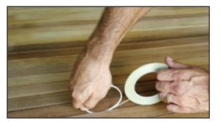
**11.** DO NOT USE PRIMER. For best results, a bond breaker tape should be applied to the bottom of a 3/16" (5 mm) or deeper seam before caulking. It prevents the caulking from adhering to bottom of the seam. A second roll of tape or the tape core can be used to guide the tape into the seam.
